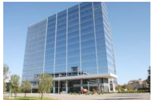
Hines' La Jolla Commons office high-rise in UTC earned U.S. Green Building Council's Leadership in Energy and Environmental Design gold status earlier this month.
